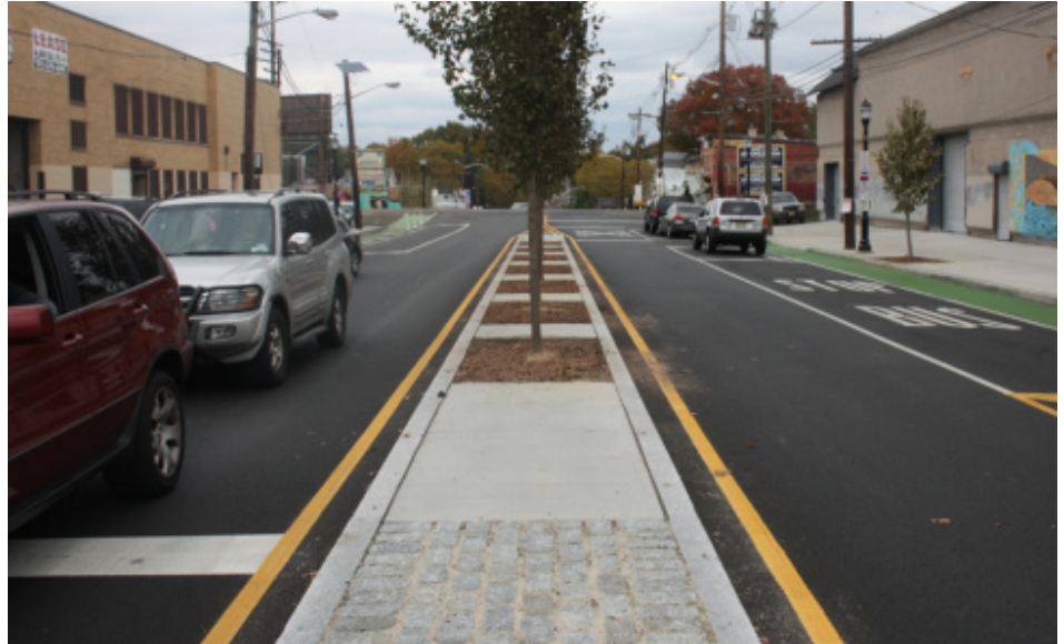
Center median located on Mt. Prospect Avenue includes granite cobbles and columnar street trees.
