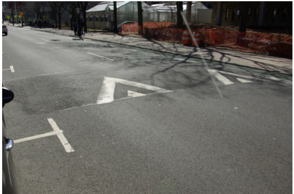
A speed hump located on University Avenue between Bleeker Street and Warren Street.
