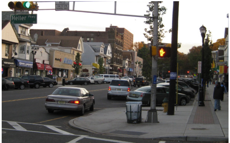
Curb extensions on Mt. Prospect Avenue significantly reduce the crossing distance by extending the sidewalk into the angled parking lane.
