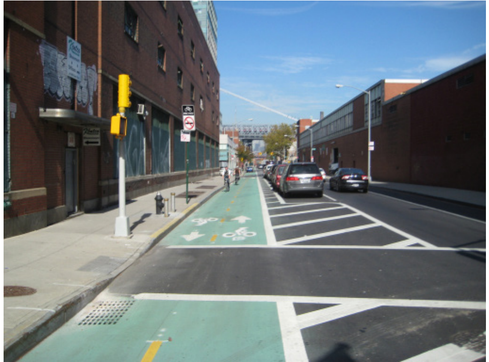
In Brooklyn, NY, the Kent Avenue two-way protected bicycle lane uses a painted buffer and off-set parking to separate the vehicle travel lane from bicyclists.
