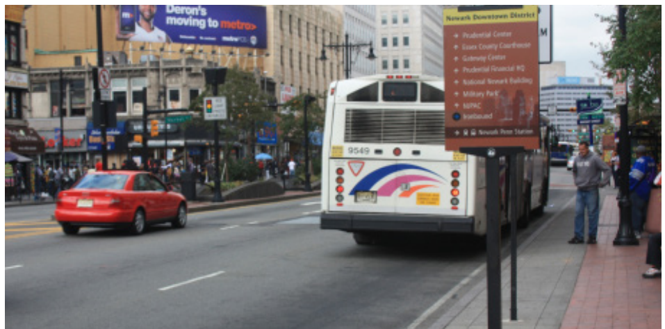
Far side bus stop where the curb was extended on Broad Street.
