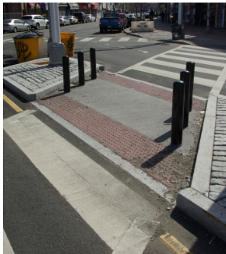
Pedestrian refuge island Bloomfield Avenue at the intersection of Broadway.
