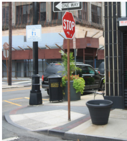
Linden Street and Halsey Street Newark Downtown District granite curb ramp.
