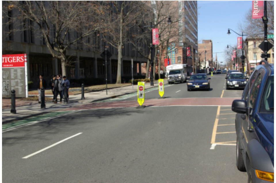
A mid-block crossing located on the Rutgers Campus on University Avenue.
