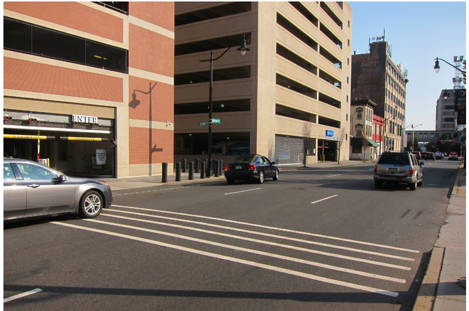
Rumble strips located on University Avenue.
