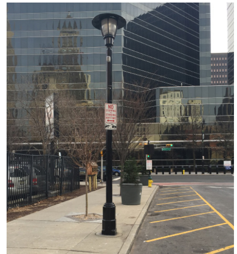
Pedestrian-scale post top fixture on Clinton Street.
