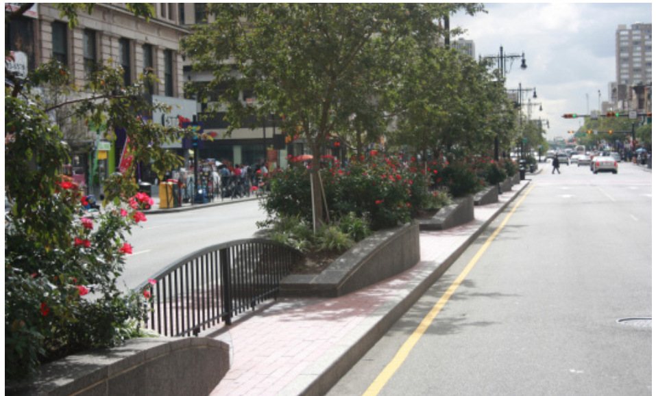
Center median located on Broad Street includes raised planters and pedestrian fences to prevent jaywalking.
