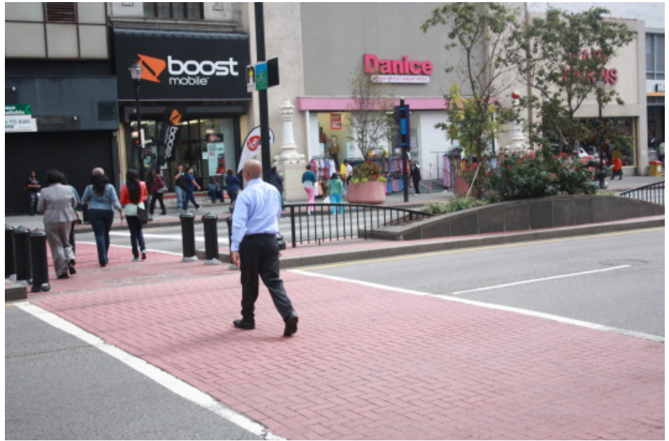
Pedestrian refuge integrated into the median on Broad Street.
