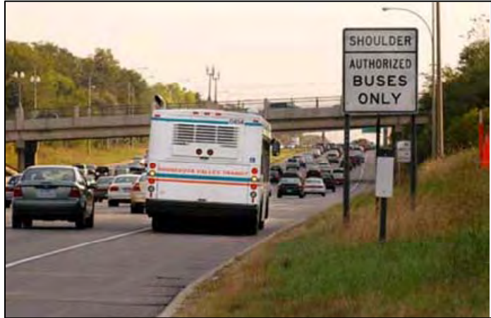
Minnesota bus shoulder lanes.
