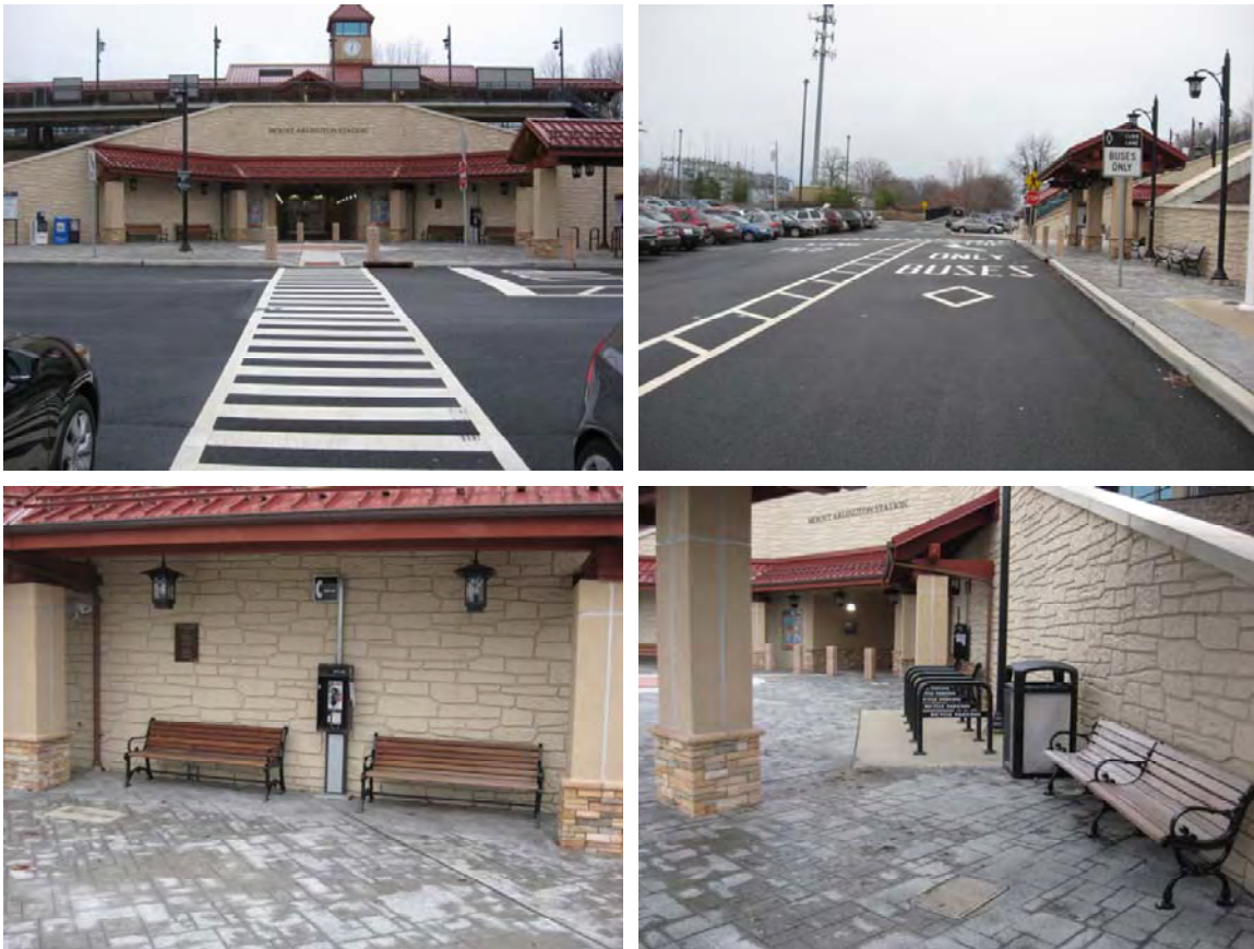
Pedestrian crosswalks, bus-only lanes, shelters, bicycle racks, benches, lighting, and trash bins
