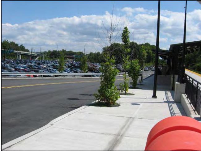
Access roadway within facility
