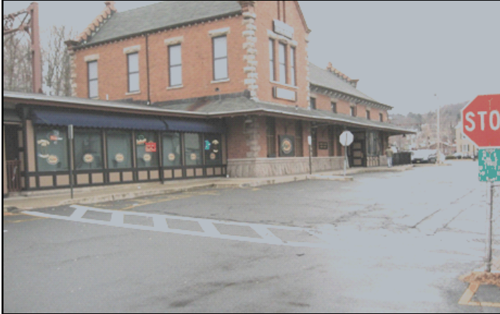
Looking west on Dickerson Street at NJTRANSIT Dover Rail Station
