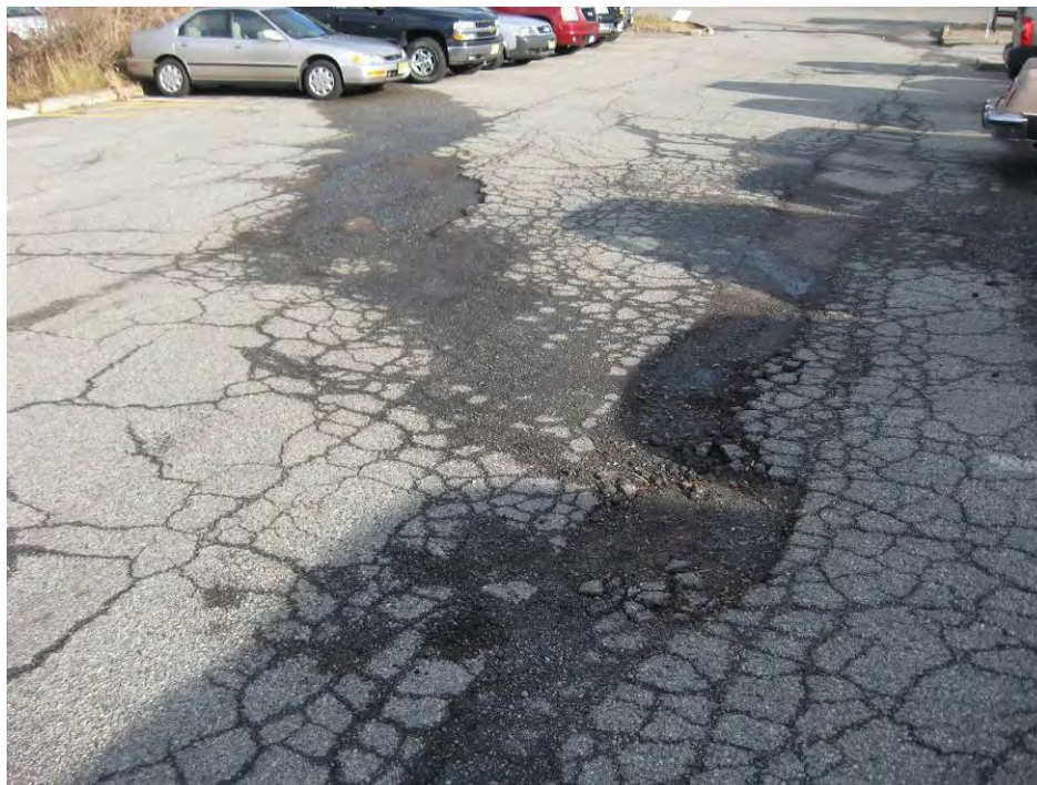
Figure 4-10: Pavement in Need of Repair (West Milford Park-and-Ride).
