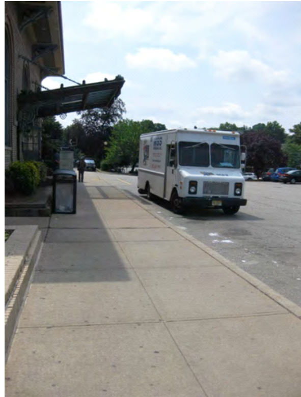
NJ TRANSIT Morristown Station building
