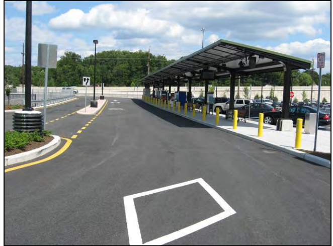
Bus-only lanes and passenger waiting area
