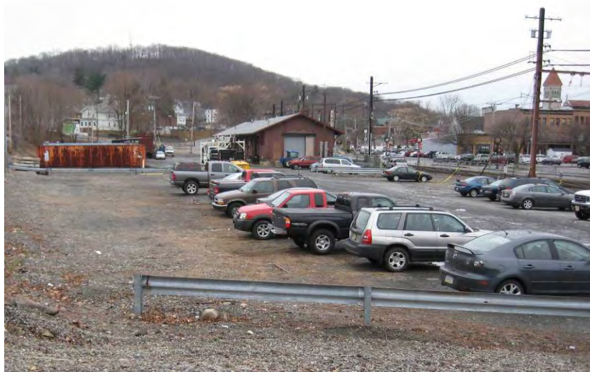
Figure 4-12: Poorly Paved Parking Lot (NJT Dover Station)
