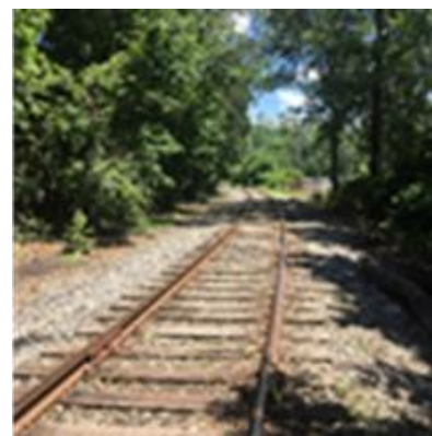
Approach to D&R Switch with NJ TRANSIT Morristown Line
