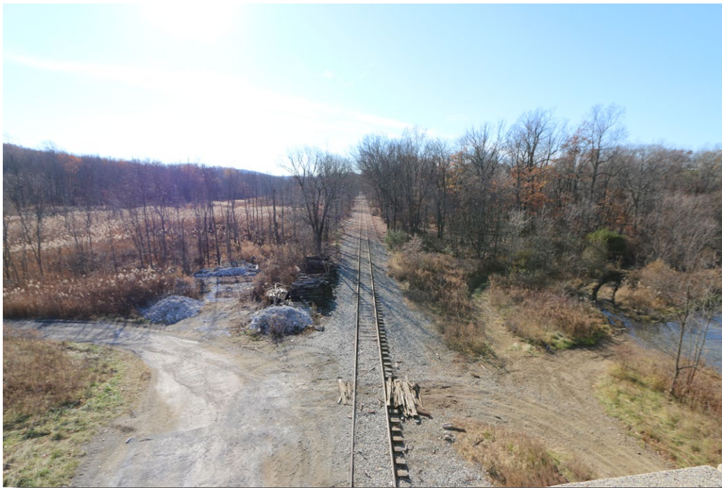
Plate 7: Overview of the Dover and Rockaway River Railroad from the State Route 46 Bridge.
