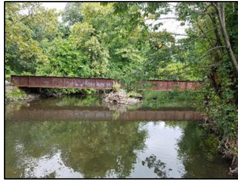
D&R Bridge over Rockaway River
