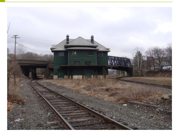
Raising the South Main Street Bridge, which will be a difficult task as it ties into existing building elevations and the old Station House, will solve the clearance issue. The current geometry, however, is low speed and the track geometry lends itself to high maintenance as the many gage rods now in the track indicate.
