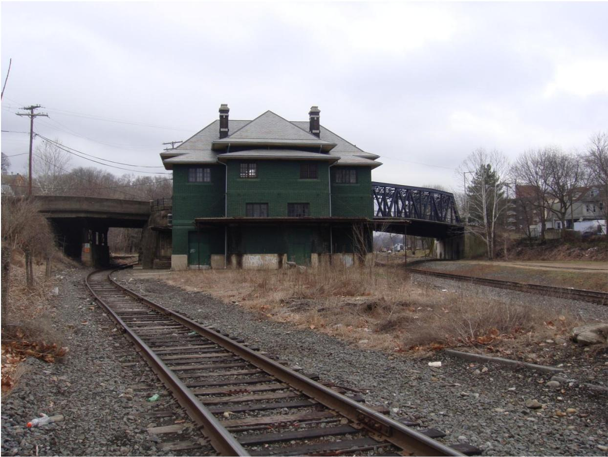
Raising the South Main Street Bridge, which will be a difficult task as it ties into existing building elevations and the old Station House, will solve the clearance issue. The current geometry, however, is low speed and the track geometry lends itself to high maintenance as the many gage rods now in the track indicate.
