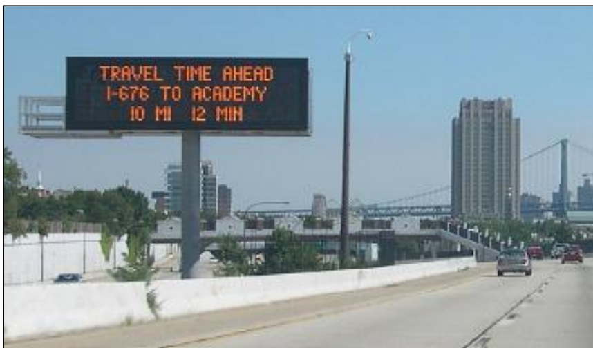
Figure 6a – Picture of Travel Time signage on I-95 in the Philadelphia area
