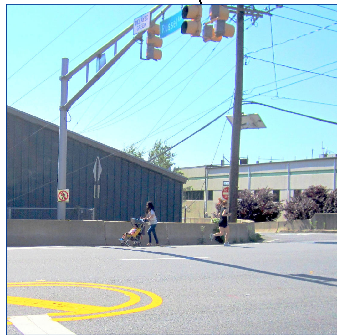
Missing sidewalk and concrete barrier requires pedestrians to use roadway shoulder
