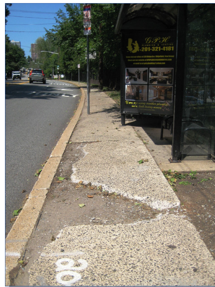
Poor sidewalk condition by bus stop
