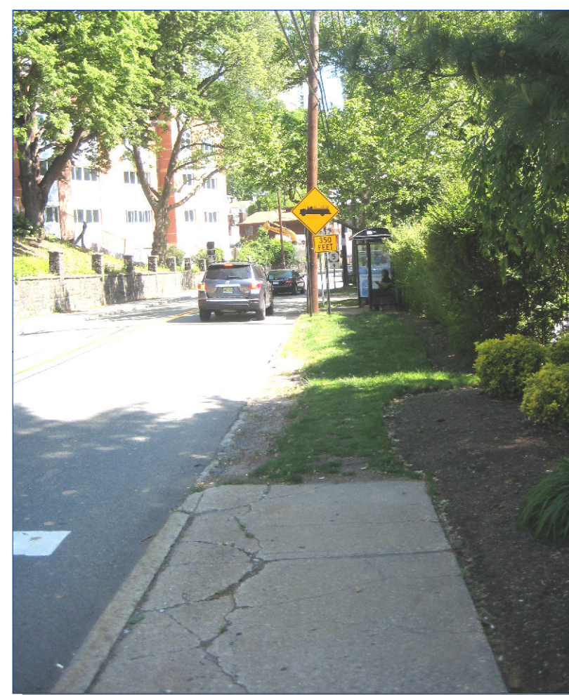
No access to bus stop due to missing sidewalk
