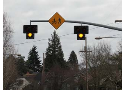
High-intensity Activated Crosswalk (HAWK signal)
