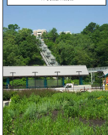
Figure 23 –Pedestrian stairwell near Port Imperial Station in Weehawken
