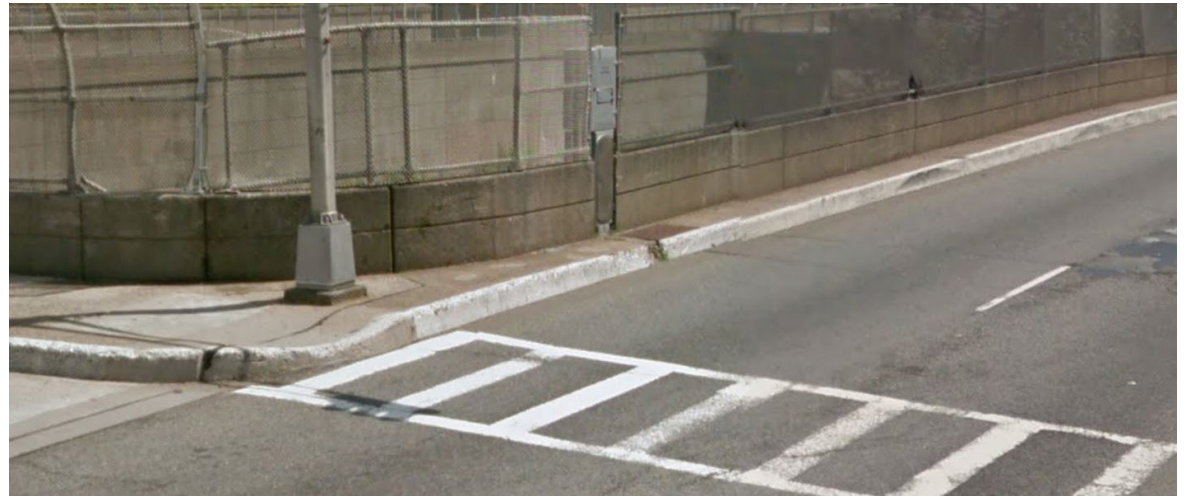
Very active crossing at Clinton Street with a four inch ramp lip
