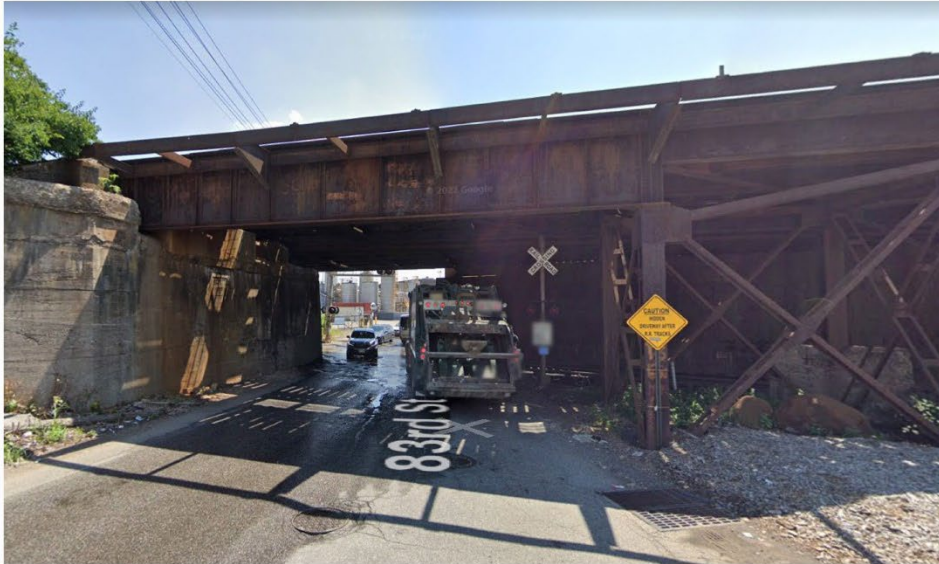
83rd Street at CSX Railroad bridge
