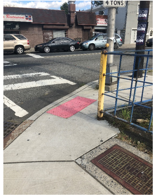
Example of a sidewalk obstruction at Danforth Avenue. Source: FHI
