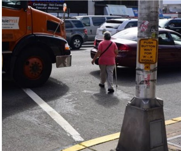
Poor pedestrian visibility was an identified deficiency at many crossings along the corridor. Hudson County has already started adding high-visibility crosswalks throughout the corridor. Source: FHI
