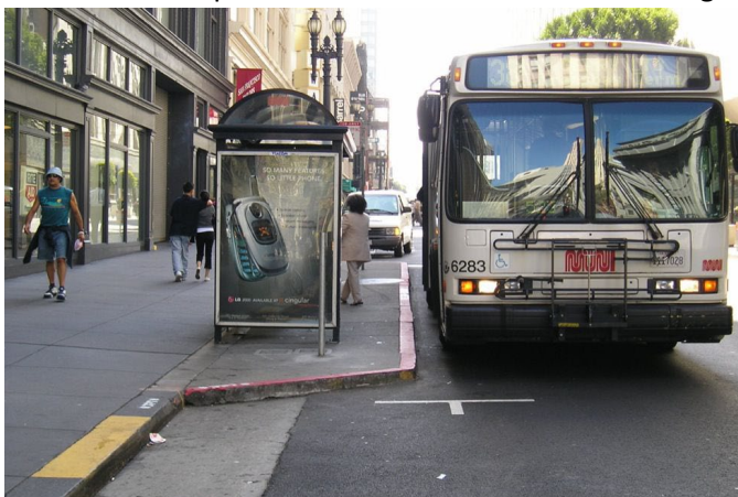
Example of a bus bulb in San Francisco. Source: NACTO
