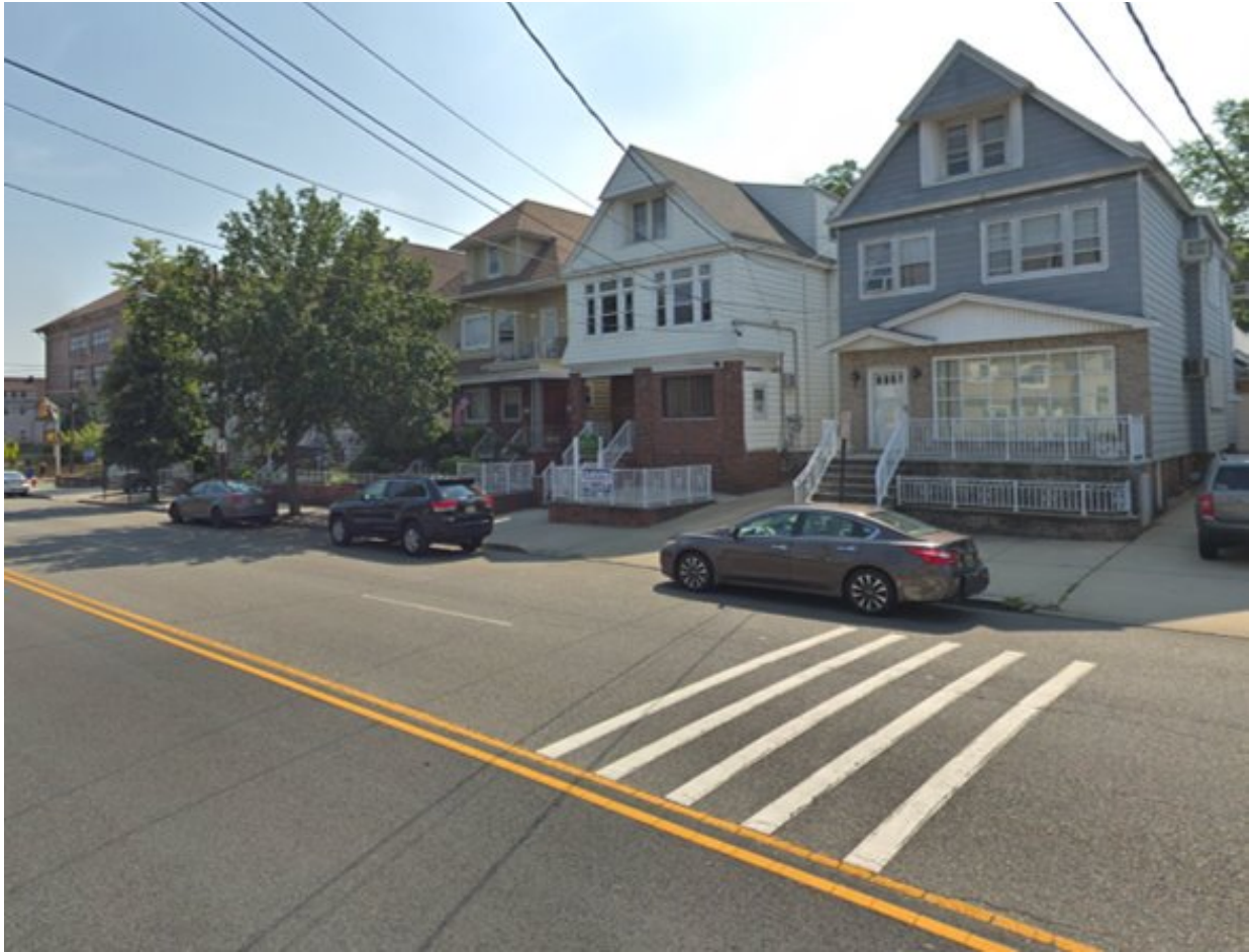
Painted rumble strips on Kennedy Boulevard are often implemented near schools. Source: Google Street View
