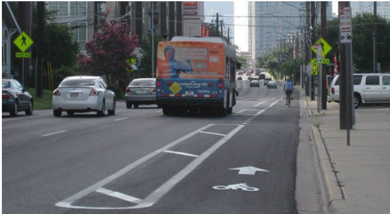
A painted buffered bike lane in Austin, Texas. Source: NACTO
