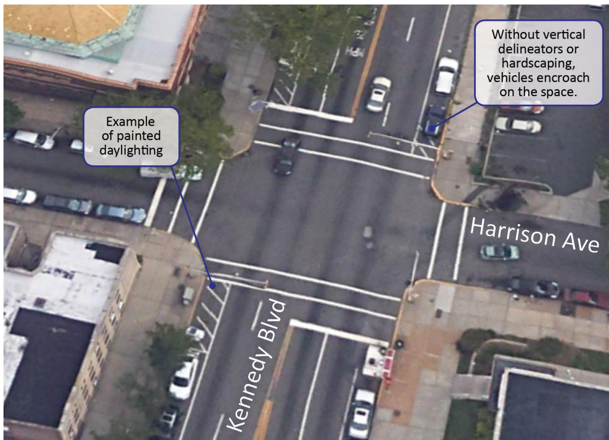
Figure 9 Daylighting on Kennedy Boulevard
