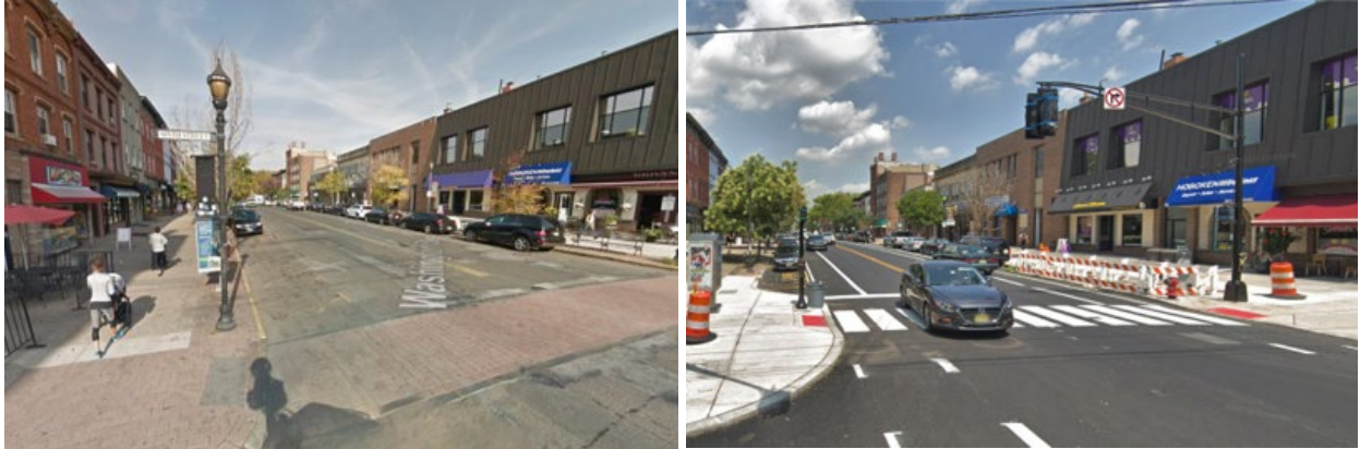
Images of Washington Street and 6 th Street in Hoboken before and after curb extensions were installed. Source: Google Street View
