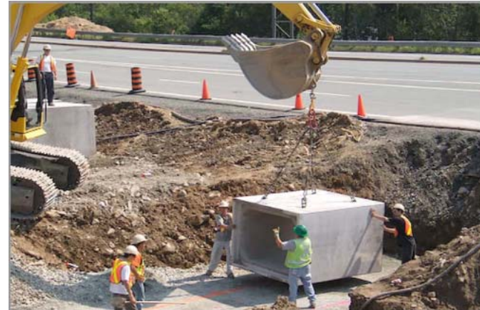
Figure 27: The installation of precast concrete box culverts of 10 feet in height and 13 feet in width can be done under the road bed, but may require the tunnel grade to be lower than the trail grade and entail drainage design that could increase costs.
