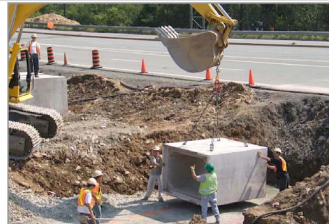
Cutoff Wall (Dowel Holes are Cast Into Floor Slab, and Reinforcing is Provided for Doweling On-Site)
