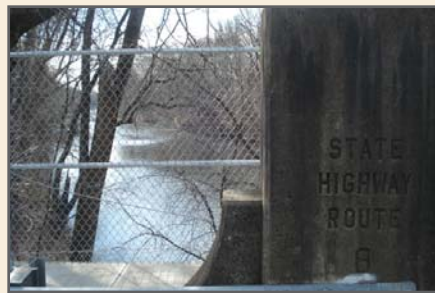
The inscription on the bridge abutment at the Passaic River crossing serves as a remnant of the New Jersey Highway 8 designation from 1917.
