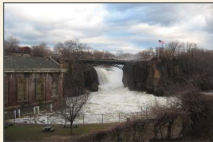
The Great Falls in Paterson and the hydroelectric plant, which was designed by Thomas Edison’s Electric Company.
