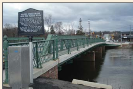
The Hillary Street Bridge over the Passaic River in Totowa.
