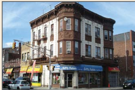
A classic mixed-use building on the corner of Market and Passaic Streets.
