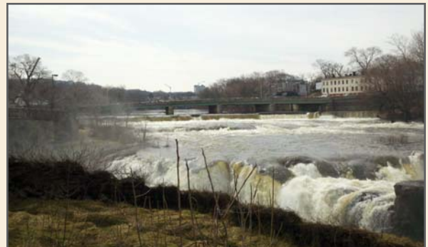
County bridges should provide pedestrian and possibly boat access to the river. Designs should take into account the surrounding context as they are rebuilt and maintained.
