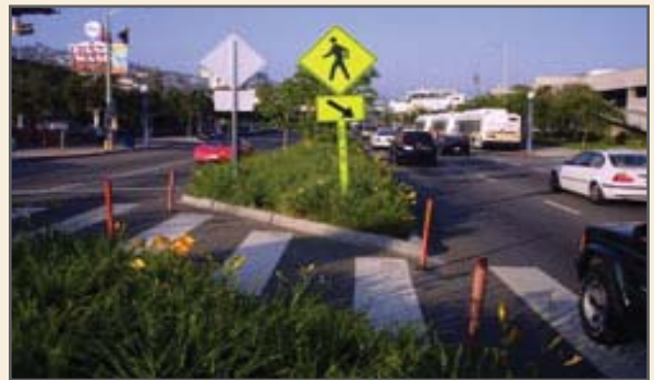
Pedestrian refuges provide a safe break at larger intersections and can help individuals with physical disabilities cross roads in a safe manner.
