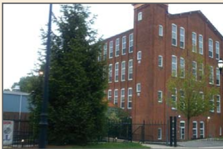
The Haledon Borough municipal building near the intersection of Church Street and Belmont Avenue.
