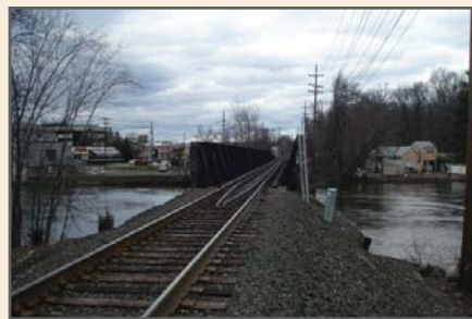
The Passaic River crossing in Little Falls.
