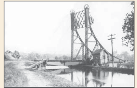
Cable-lift bascule bridge with curved-track rolling counterweight, formerly at Mountain View, Wayne.
