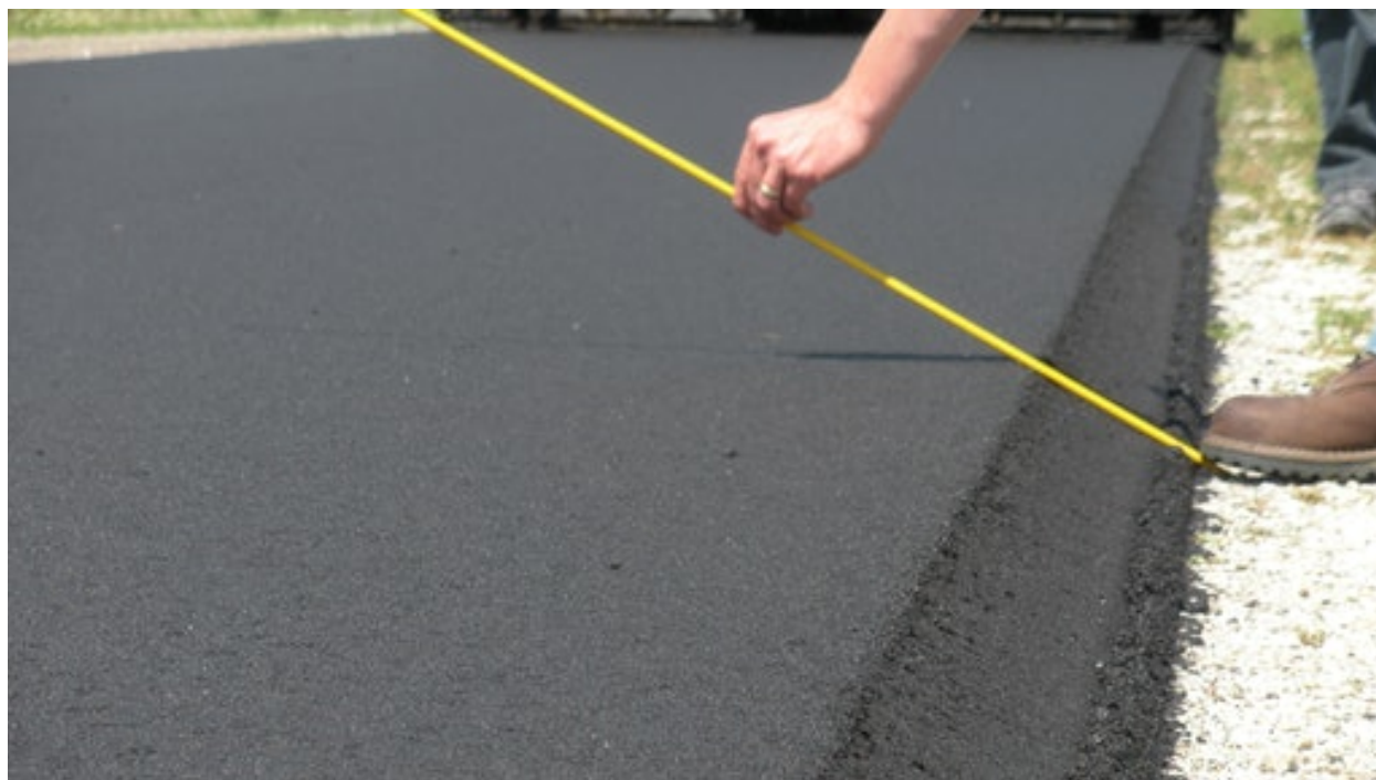
Figure 16 – Safety Edge Paving Example 23
