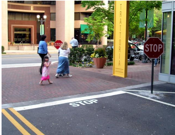
This sidewalk’s brick texture makes it stand out to the driver and is reinforced with a stop sign.
