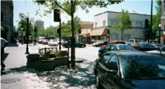
This curb extension has been landscaped, adding to the traffic calming effect by narrowing the field of vision vertically as well as horizontally.
