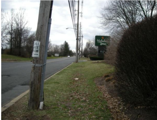
A footpath along Davidson Avenue indicates the need for sidewalk installation to better serve workers on this corridor.
