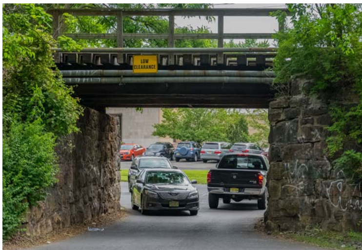
Narrow one-lane underpass of the NJ TRANSIT Raritan Valley Line along Milltown Road, near its intersection with Doolittle Drive
