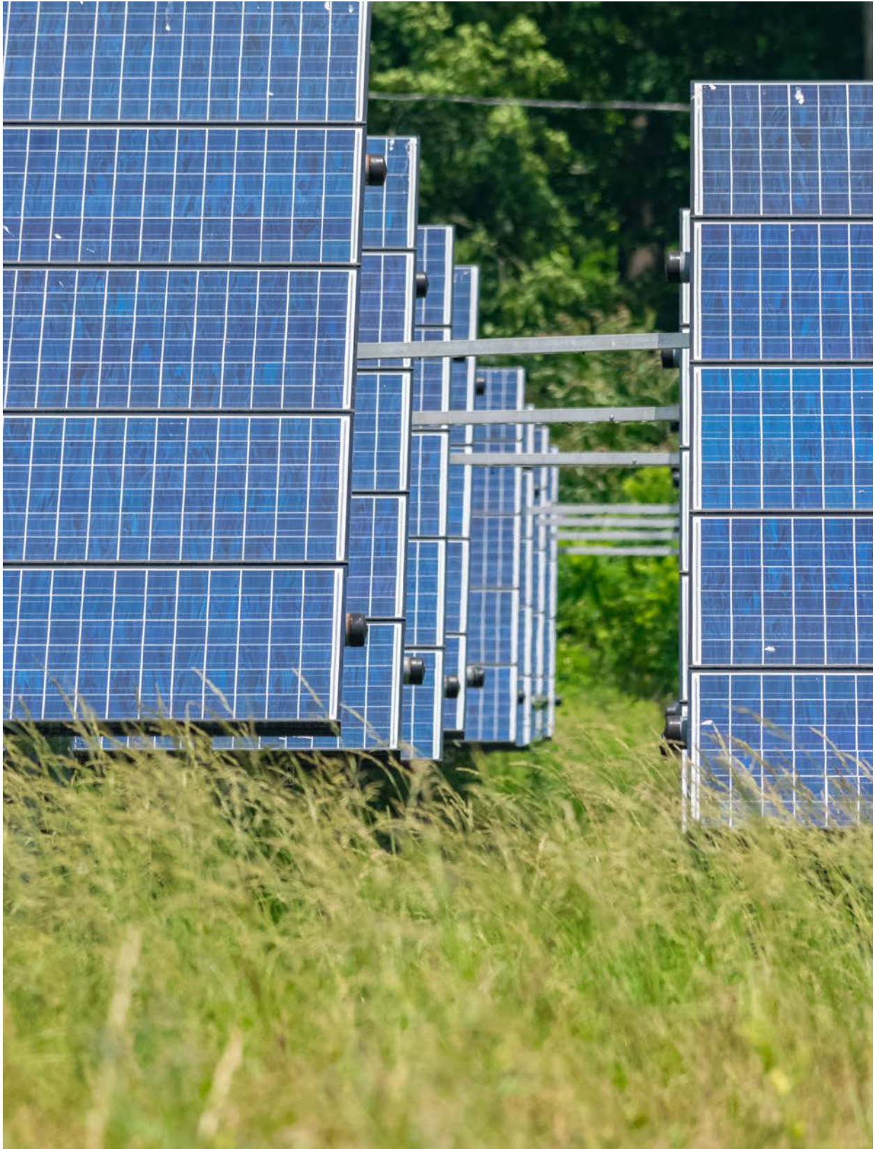
Solar array at Duke Farms in Hillsborough
