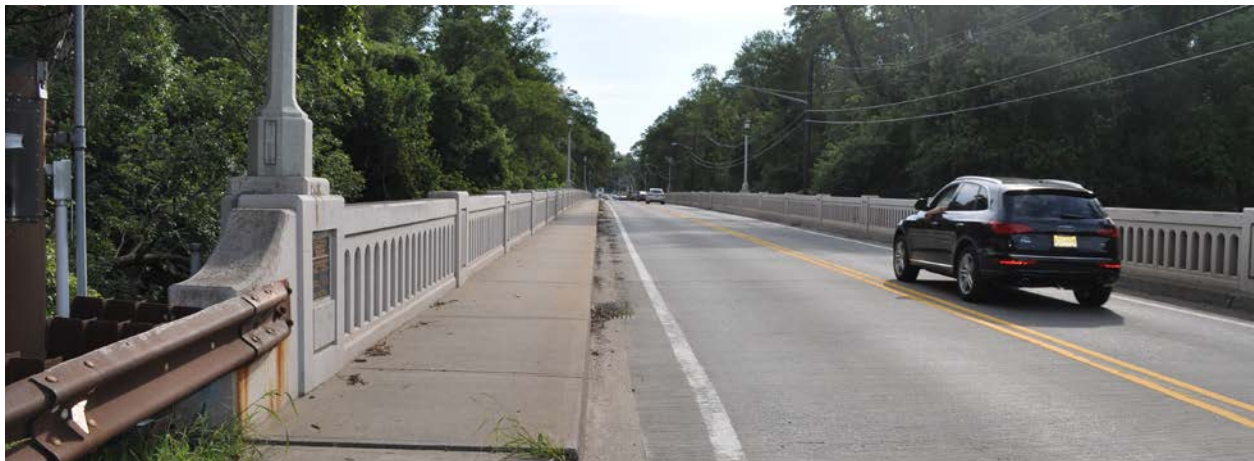
Existing CR 514 causeway is too narrow to accommodate a bicycle facility
