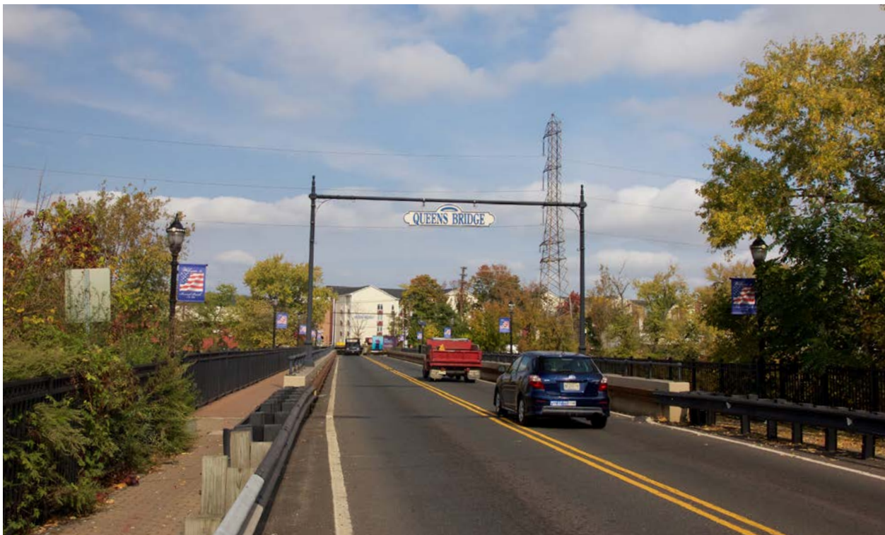
The Queens Bridge, connecting South Bound Brook and Bound Brook over the Raritan River
