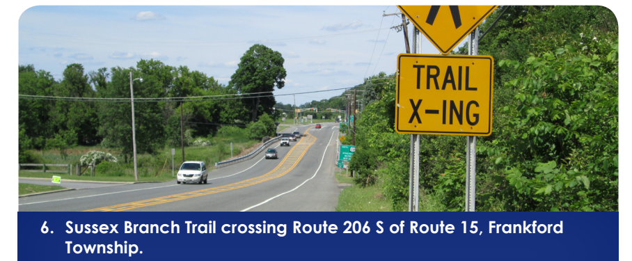
6. Sussex Branch Trail crossing Route 206 S of Route 15, Frankford Township. Warning trail crossing signs on roadway. No painted crosswalk or signs where the trail actually crosses roadway. High-speed traffic and poor sight distance approaching from south (vertical alignment – hill) exists.
