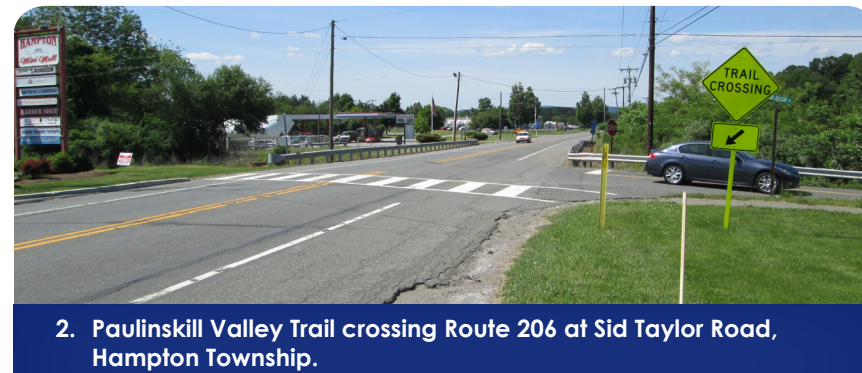
2. Paulinskill Valley Trail crossing Route 206 at Sid Taylor Road, Hampton Township. Signage alerting drivers that they are approaching a trail crossing is located on Route 206. There is a painted crosswalk at the trail crossing. High-speed traffic is typical along this stretch of Route 206.
