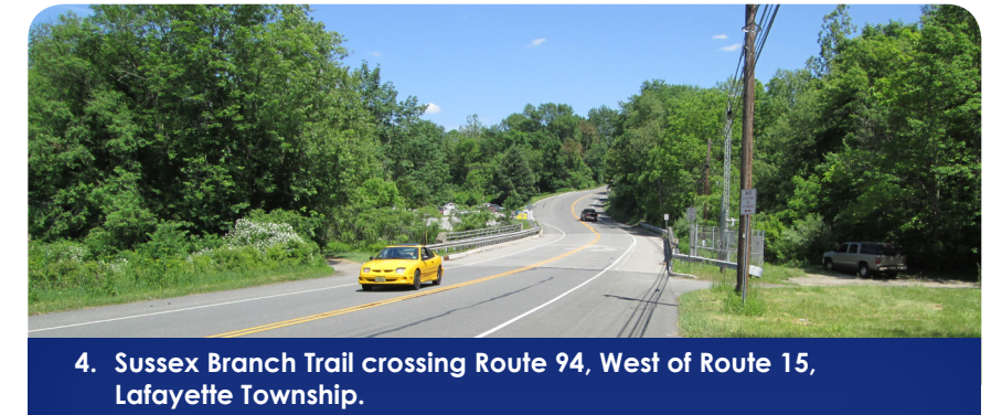
4. Sussex Branch Trail crossing Route 94, West of Route 15, Lafayette Township. Trail parking areas are provided, but no trail crossing signage or crosswalks. The roadway curves and traffic is moving downhill in both directions toward the trail, causing visibility issues and resulting in fast-moving traffic.
