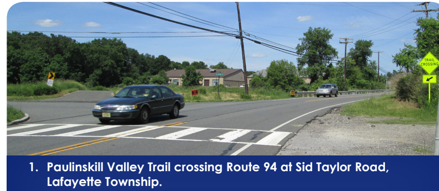
1. Paulinskill Valley Trail crossing Route 94 at Sid Taylor Road, Lafayette Township. Route 94 has signage alerting drivers that they are approaching a trail crossing. This trail crossing has a painted crosswalk. The sight distance is poor for motorists approaching the trail crossing.
