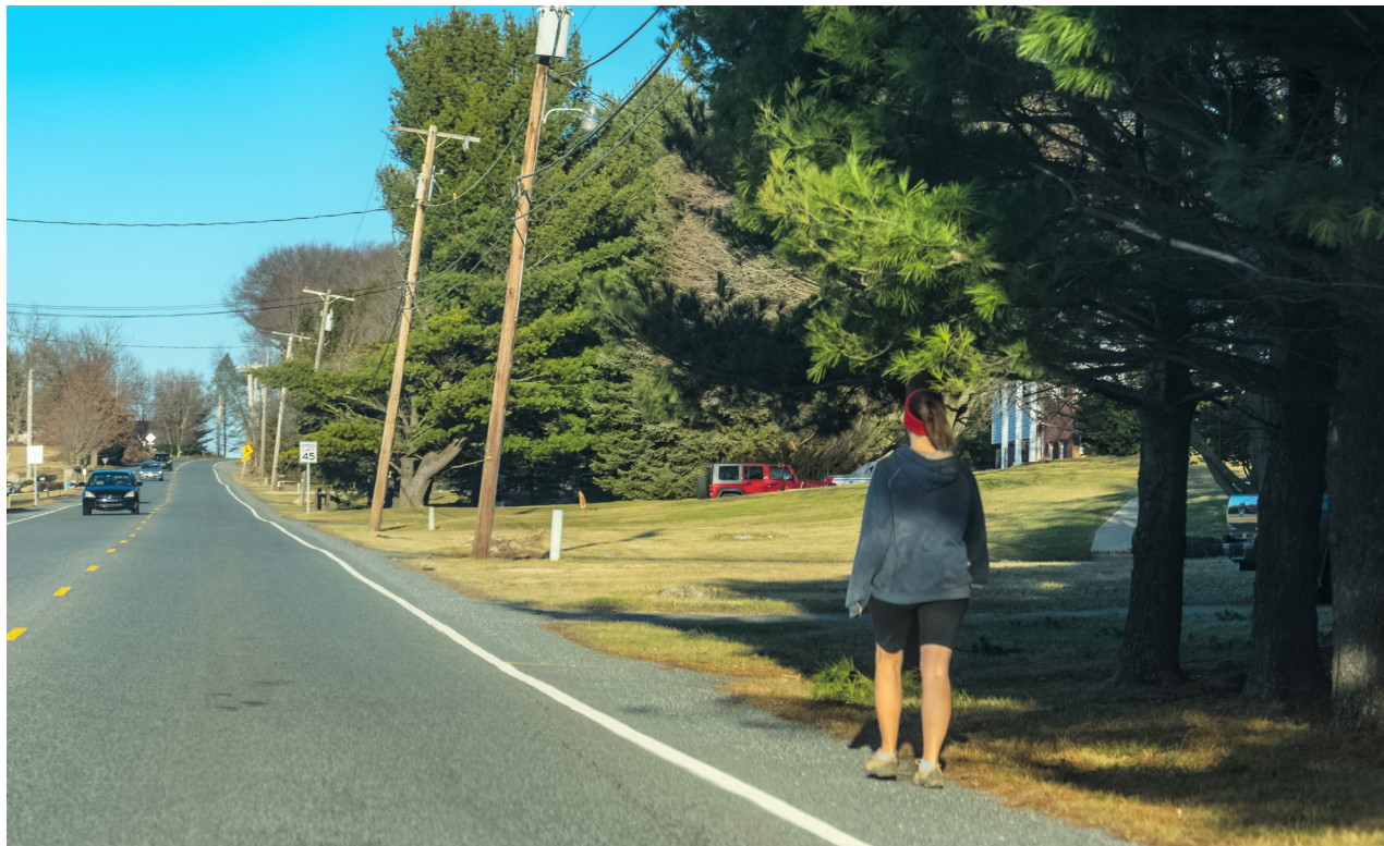
Many Rural roadways in Warren County lack adequate pedestrian accommodations
