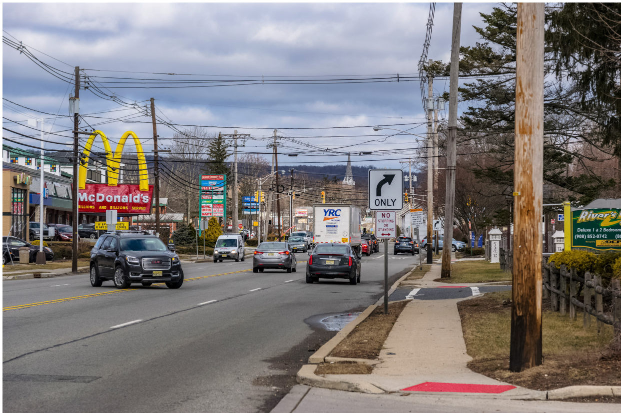
Outdated strip commercial development and roadway design contribute to chronic peak hour congestion on Mountain Avenue (NJ 182) in Hackettstown
