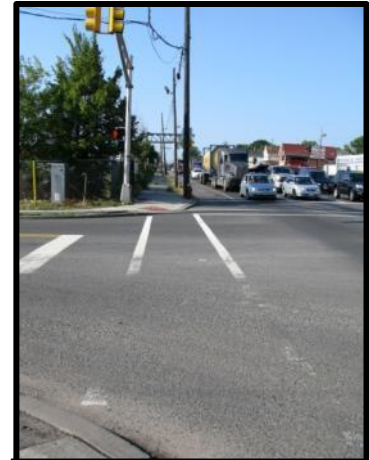
Worn striping typical of entire Route 1&9 Corridor
