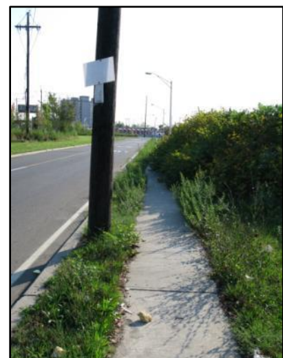
Poor Maintenance along sidewalk at North Avenue
