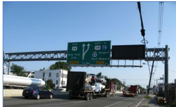
Route 1&9 Northbound north of Fairmount Avenue, approaching the transition to the freeway portion of Route 1&9
