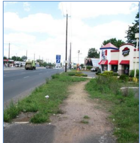
Route 1&9 Northbound between Milton Avenue and Patterson Street. The heavily worn path indicates significant pedestrian traffic along this gap in the sidewalk network.
