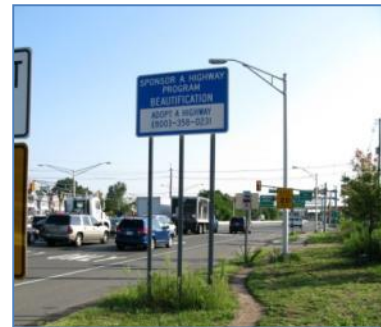
Route 1&9 Northbound approaching North Avenue looking north. The heavily worn path indicates a gap in the sidewalk network approaching an existing bus stop
