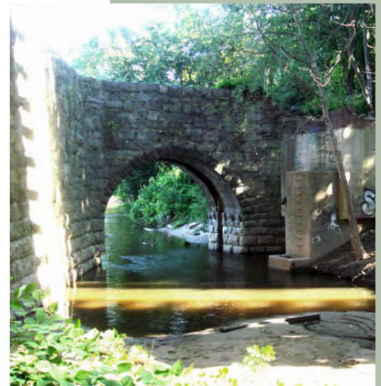
Morris Canal Arch
