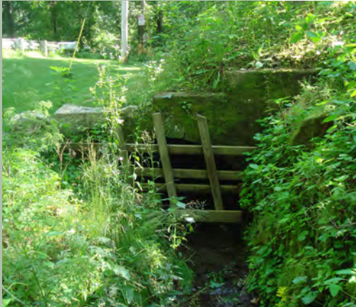
Tailrace and location of the power house of Plane 10W
