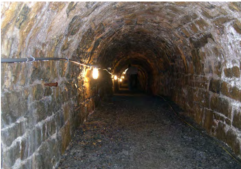
Looking up the tail race towards the Scotch turbine at Plane 9 West
