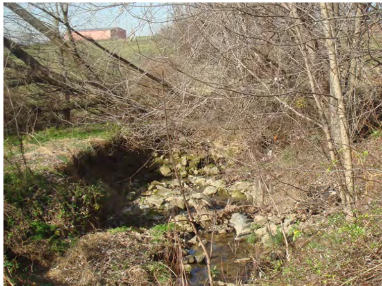
Tributary of the Lopatcong Creek erodes the canal bed just west of Strykers Road
