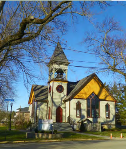
Port Colden Methodist Church
