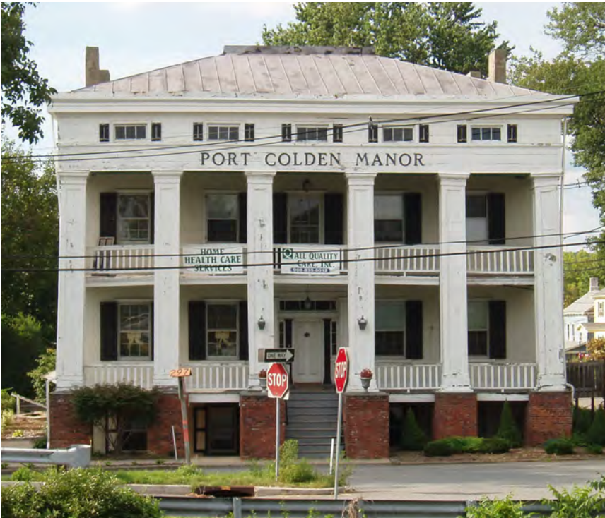
Port Colden Manor is a historic canal related structure in need of significant repair.
