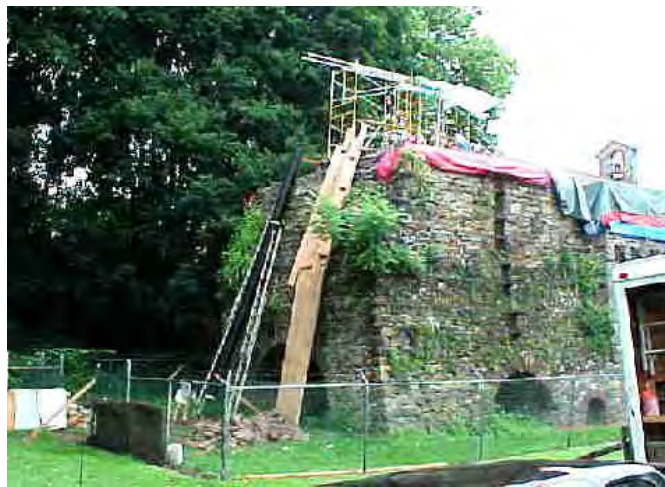
Oxford Furnace in mid-restoration Photo courtesy the Warren County Cultural and Heritage Commission
