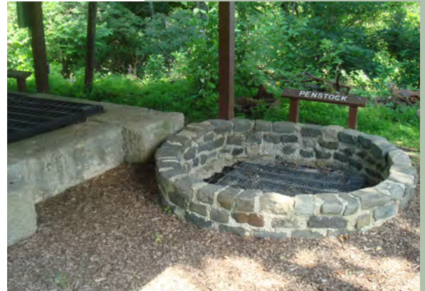
Foundation of the penstock at Plane 9W
