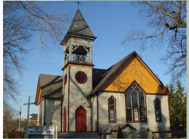
Port Colden United Methodist Church
