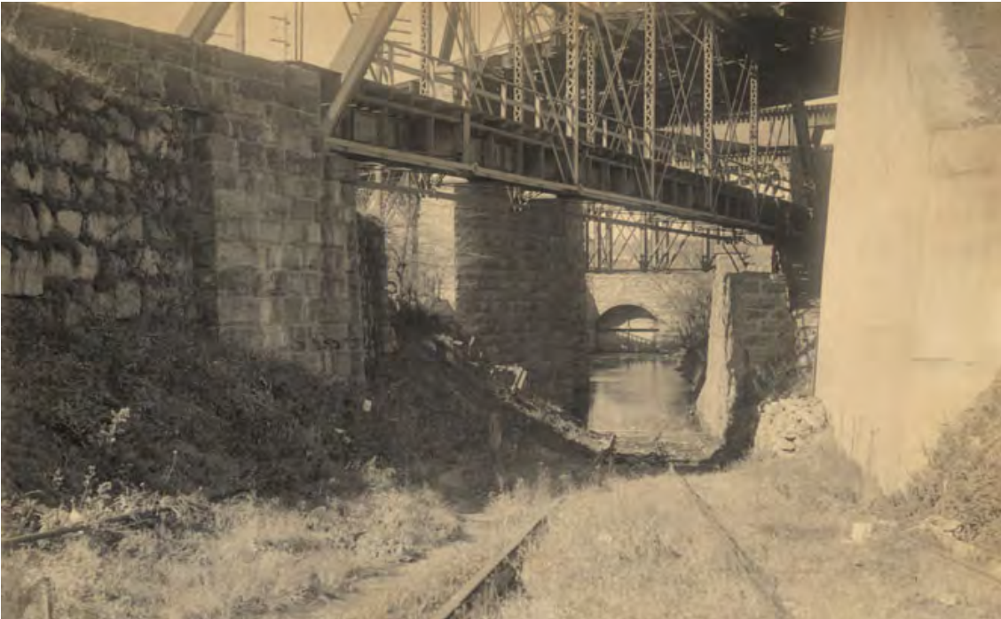
The Canal Arch in Phillipsburg represents the historic beginning point of the Morris Canal. Photo courtesy New Jersey State Archives
