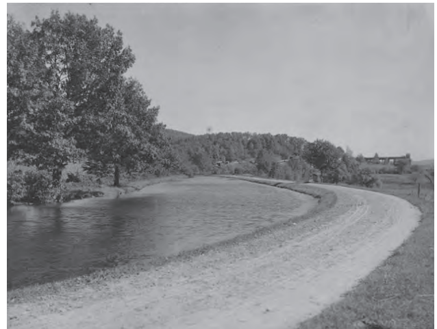
Canal near Port Colden with Plane 6 West in background Photo courtesy of NJ State Archives
