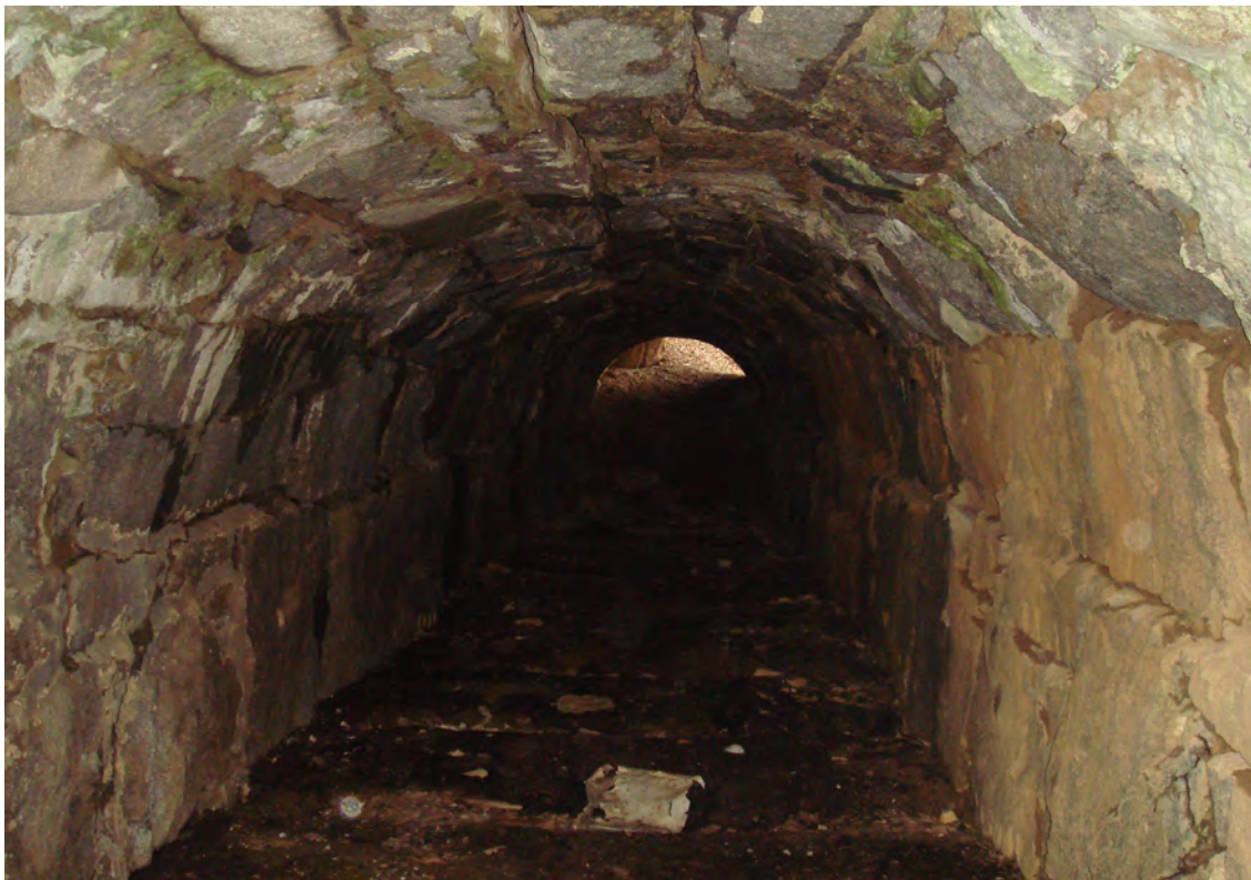
Looking down the tailrace at Plane 5W, also known as the Brickyard
