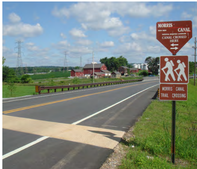
Midblock crossing at Strykers Road
