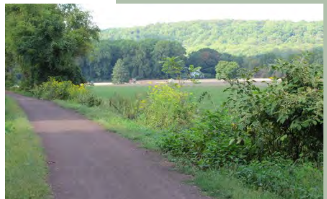
Crushed aggregate on the Delaware Canal towpath
