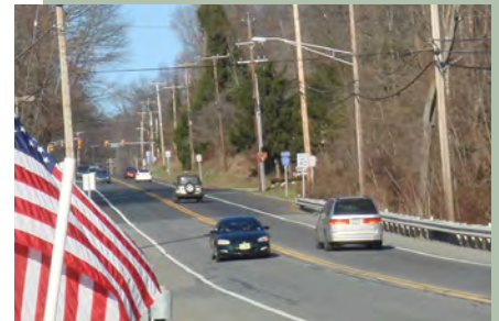
Canal crossing Route 517 near the M&M Mars plant.
