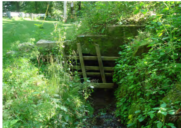
Tail race of Plane 10W is still visible along Lock Street
