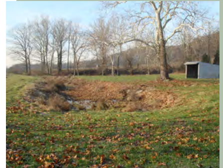
View of the canal prism from Little Philadelphia Rd.
