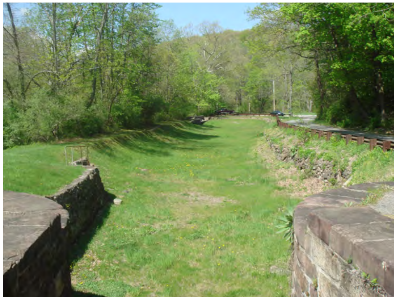
The canal prism near and remaining portions of the lock at Saxton Falls
