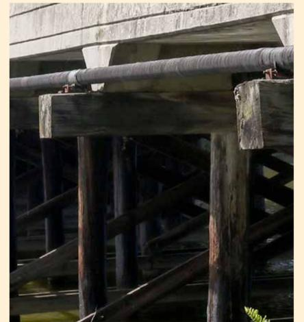
reconstructed, and the wooden bridge deck was replaced with concrete, though most of the bridge's original wooden structure was maintained. About 3,500 vehicles travel over the bridge daily. The bridge is a regional transportation link, providing motorists, pedestrians and bicyclists with access to the Allenhurst NJ TRANSIT station. It is also critical to the vitality of downtown Allenhurst. Motorists use the bridge to access nearby State Routes 35, 66 and 71.
