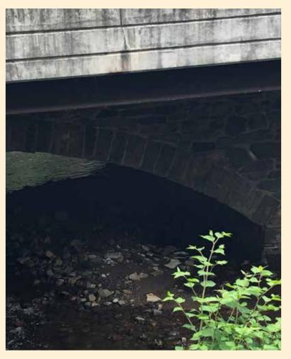
of rehabilitations and additions over the years. In 1890, a steel stringer sidewalk was added to the east side. The west side of the bridge was widened with concrete in 1908. There were additional widening and rehabilitation projects in 1964 and 1993. About 7,300 vehicles cross the bridge daily. The bridge is located near two schools, the public library, police department, a fire station and local businesses.
