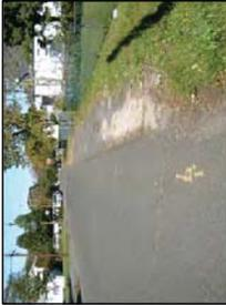
Broken sidewalk in NW corner of Hamilton St and Franklin Blvd due to truck turns
